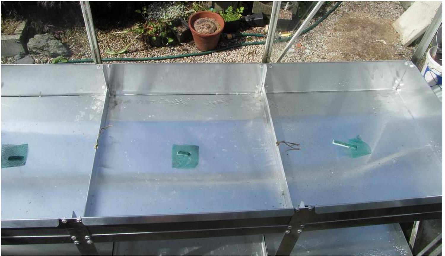
For drainage I cut a 20mm hole in the centre of each of the base sections, through this I fed a strip of capillary matting then covered the hole with plastic mesh that would prevent the sand from escaping.
