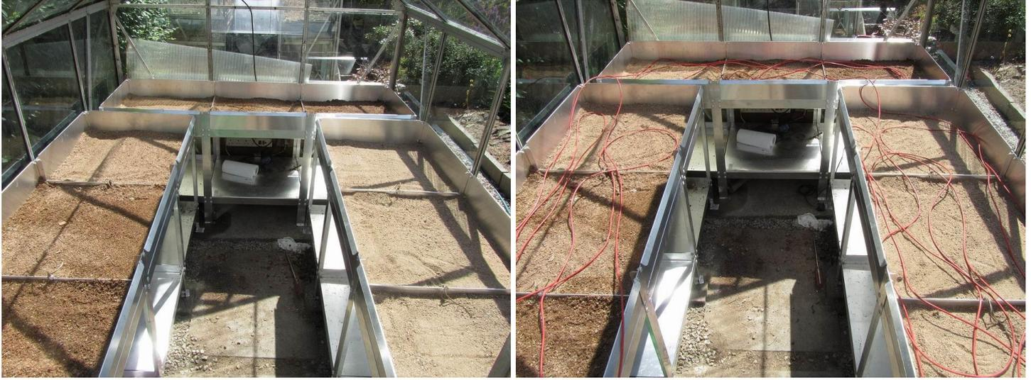
After laying around 20mm of sand I spread out a soil warming cable this is not to warm the bulbs but to protect against the sand freezing around the roots and base of the bulbs, which for some types is fatal. The cables are controlled by a thermostat and sensor placed just above the cables. This is set to come on when the temperature at that depth falls to 0C and it goes off again when the temperature rises to 2C.
