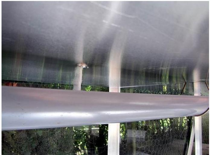
I hung plastic guttering underneath to catch the surplus water draining away and collected it in a bucket for recycling.
