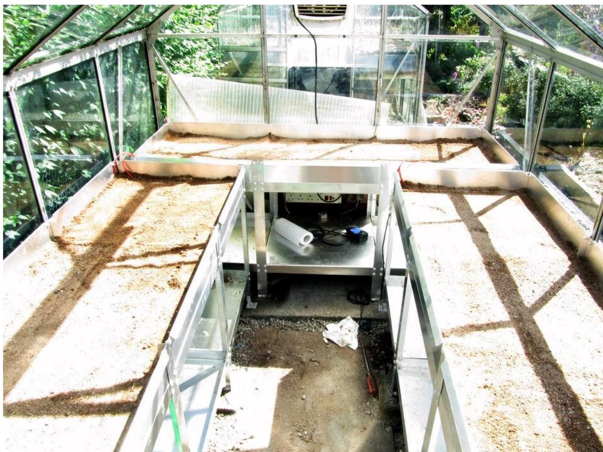
the heat wave we are having that was not a problem – on previous occasions I have to plug the cable in to warm it up and make it flexible. I roughly lay the cable so that each tray has an even distribution as shown above then I carefully space the cables in each section holding it in place by adding sand. I add a final layer of sand and level it off ready to receive the plastic pots.
